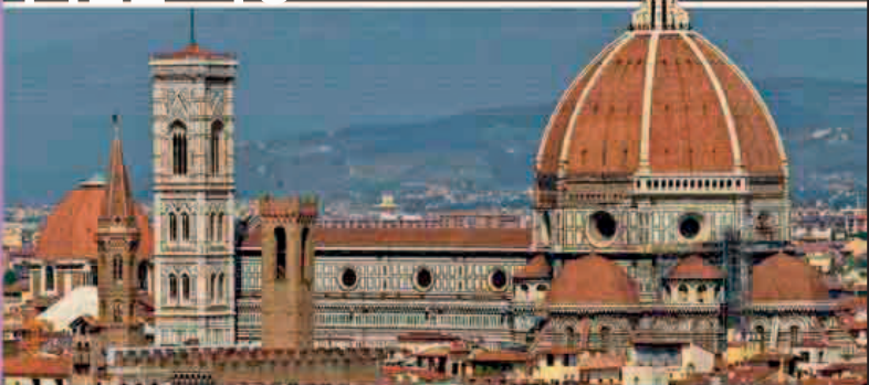
The dome of Santa Maria del Fiore cathedral, Florence, is 137.8 ft (42 m) in diameter and 171 ft (54 m) high and took its architect, Brunelleschi, 16 years to complete.
