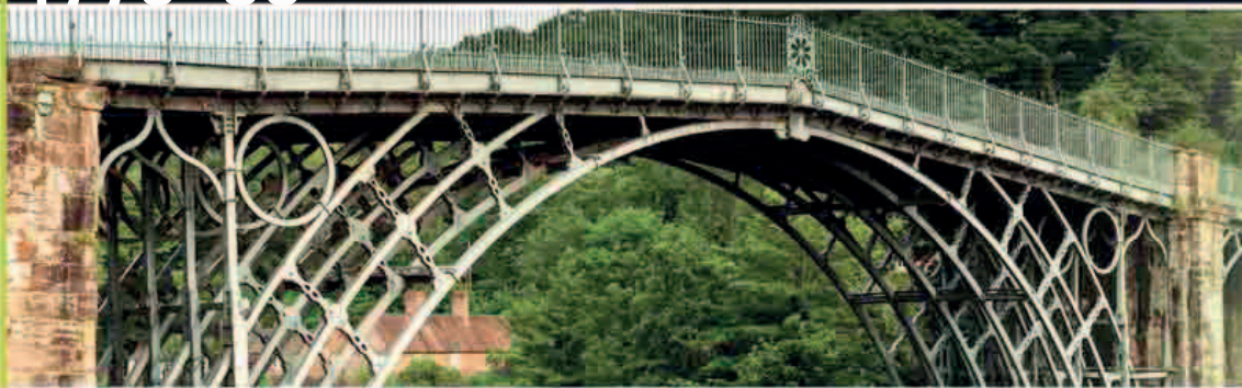
Designed by Thomas Pritchard and built by Abraham Derby III, the bridge at Ironbridge, which crosses the Severn River in Shropshire, England, was fabricated entirely from precast pieces of iron.
