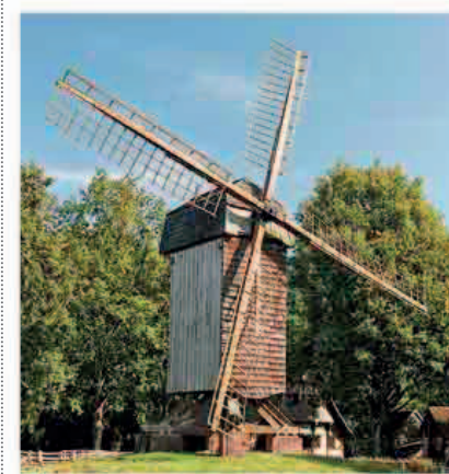
Vane power This German windmill shows the typical arrangement of four sails attached to a vertical post, but unlike earlier post-mills only the cap of the mill rotates to face the wind.
