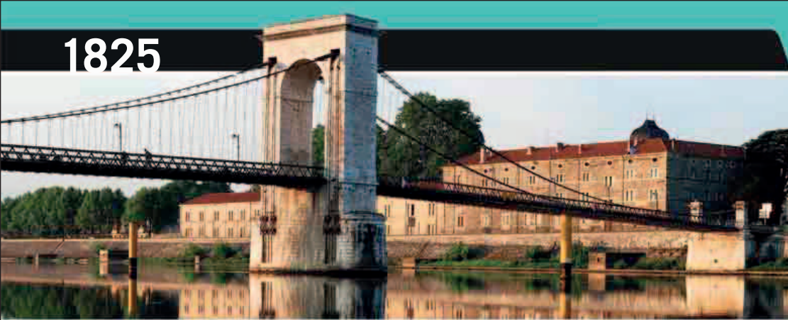
Marc Seguin's bridge across the Rhône between Tournon-sur-Rhône and Tain-l'Hermitage used a pioneering wire cable suspension system.
